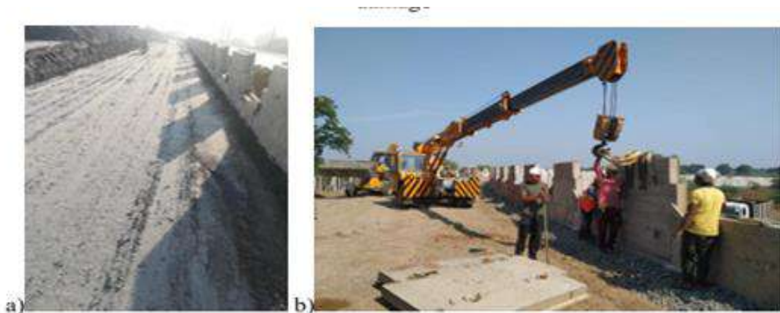
Figure 21: Typical initial course pre-cast panel placement operation
