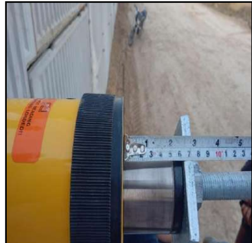
Photo No 7: Measurement of Displacement
