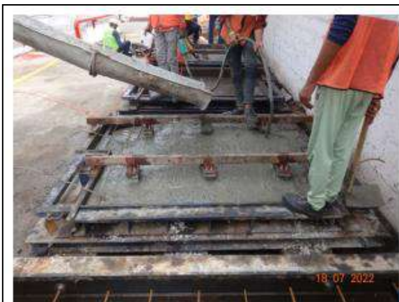
Figure 5: Compacting concrete using vibrator
