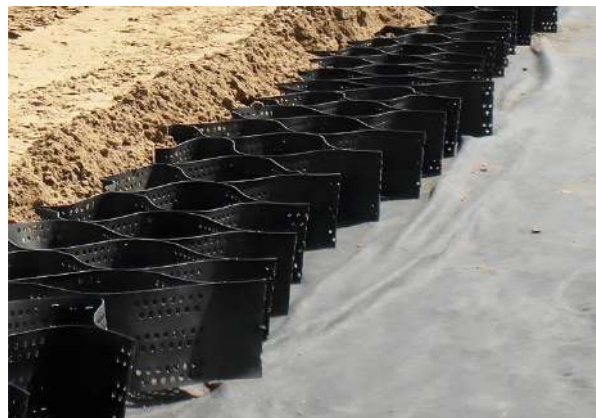
Figure 14: Geocell Basal Reinforcement (Prefabricated/Factory made Geocells)
