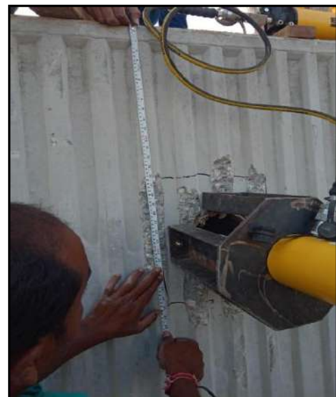
Photo No 5: Measurement of Backfill thickness above Geostrip.
