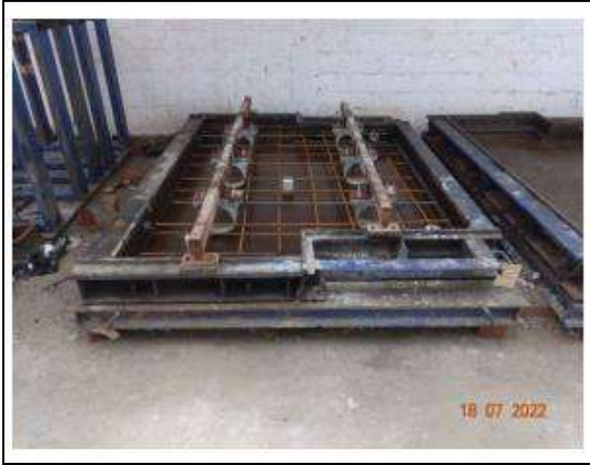
Figure 2 Panel reinforcement and connector placement witness
