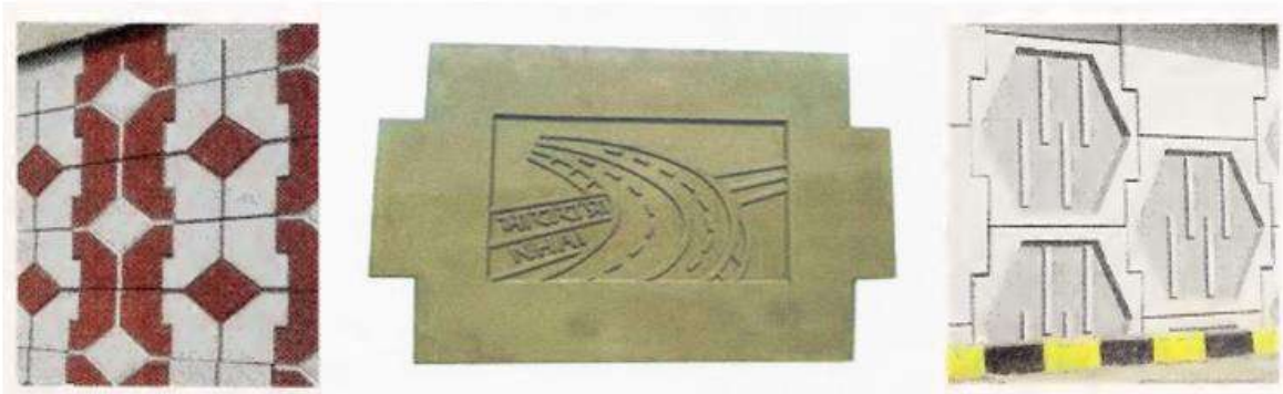
Figure 9: Panels with Architectural Finish
