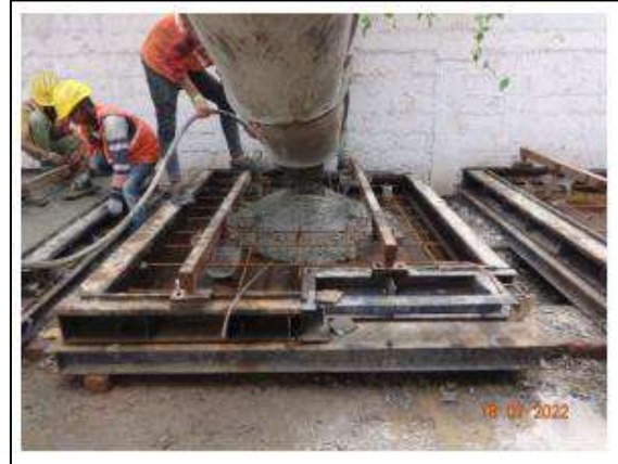
Figure 3 Concrete pouring into steel moulds
