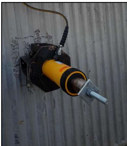
Photo No 4: Positioning of Jack and stand on hole
