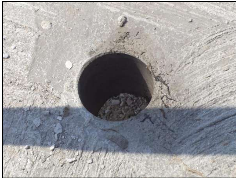
Photo No 2: Panel with 160mm diameter Hole.
