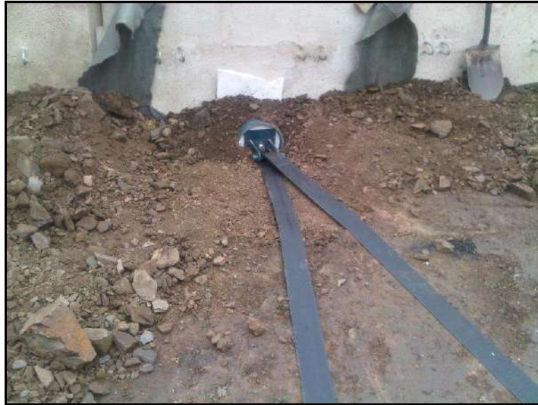
Photo No 3: Geostrip Installed for test.
