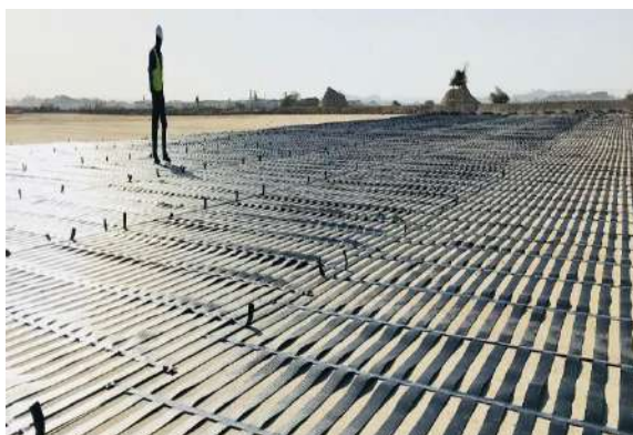
Figure 15: Geogrid Basal Reinforcement
